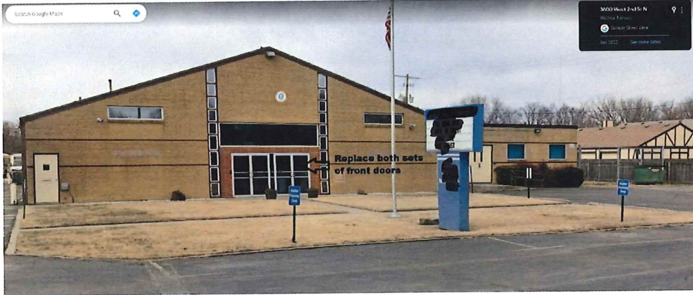
Exterior South View of Church: Figure 2. Front side of church showing the two sets of doors to be replaced.
